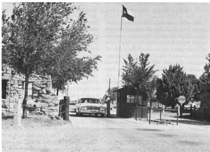
Fig. 21. The entrance gate to Palo Duro Canyon
